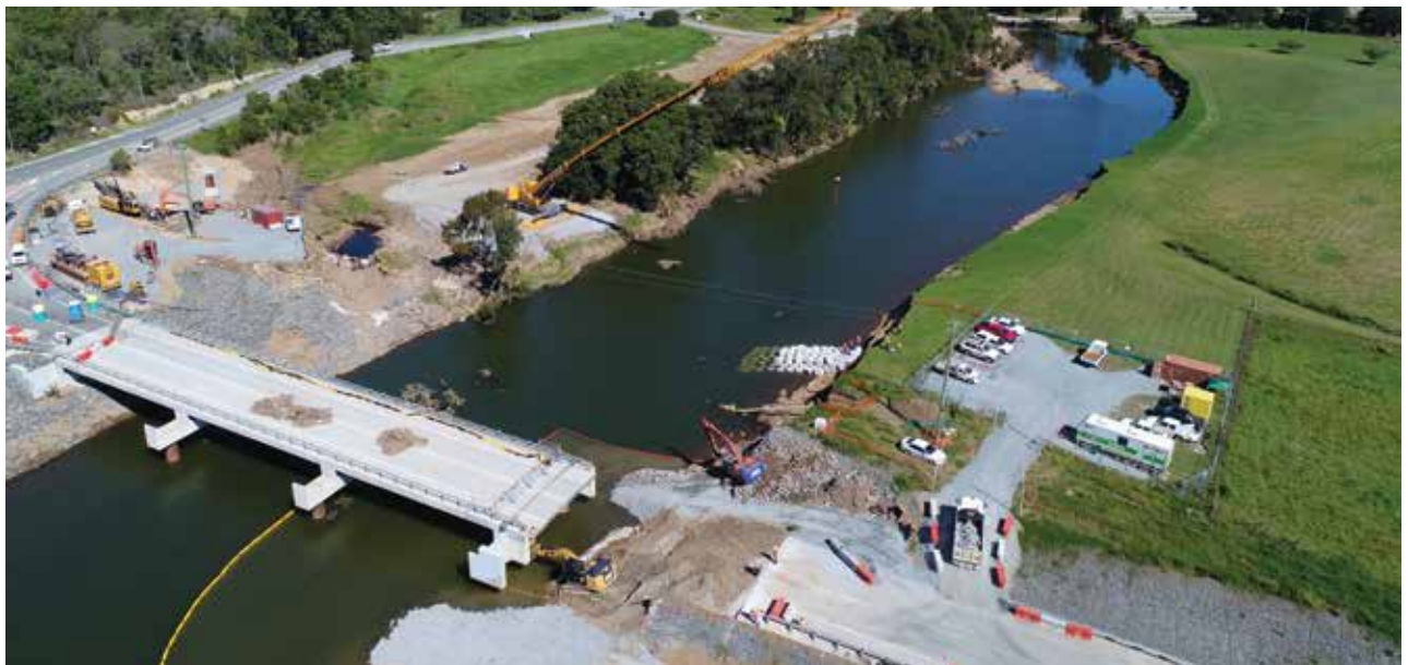
John Muntz causeway remedial works underway
