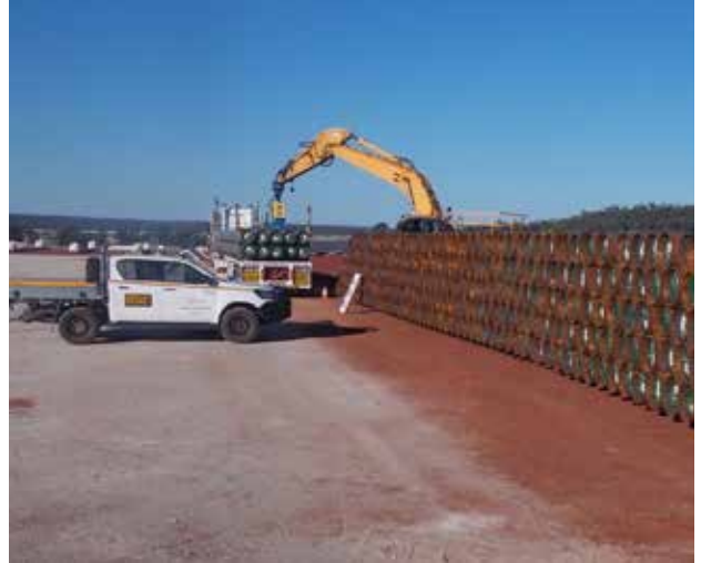
Pipe stockpile at the new Reedy Creek Wallumbilla Pipeline project
