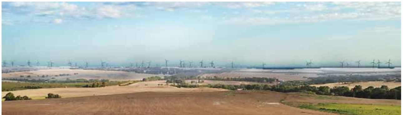
Badgingarra Wind Farm site (Emu Downs Wind Farm in the background)
