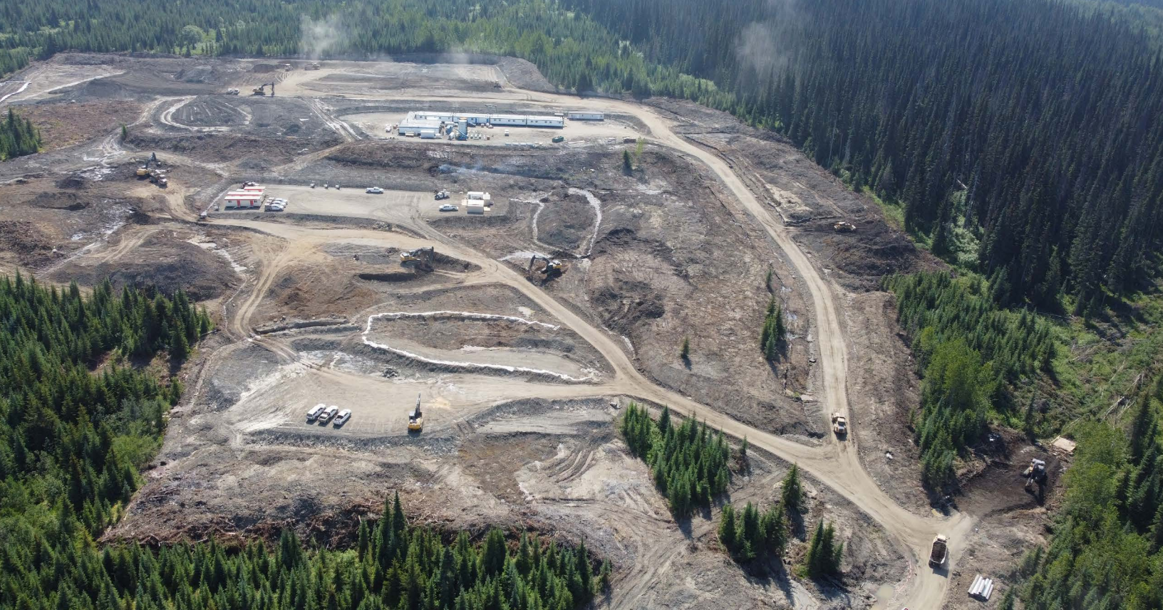
Construction in progress at KSM's Camp 11 ▲
