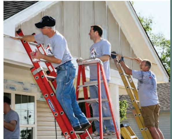
Employee House Build
