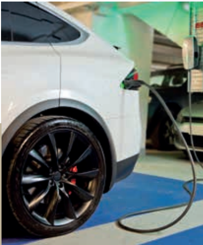
Electric Vehicle Charging at CitiPark
