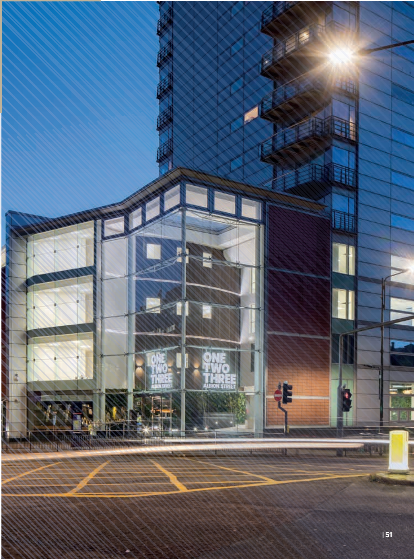
123 Albion Street, Leeds
