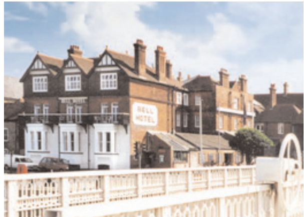
The Bell Hotel in Sandwich recently acquired by The Place Sandwich VCT Limited
