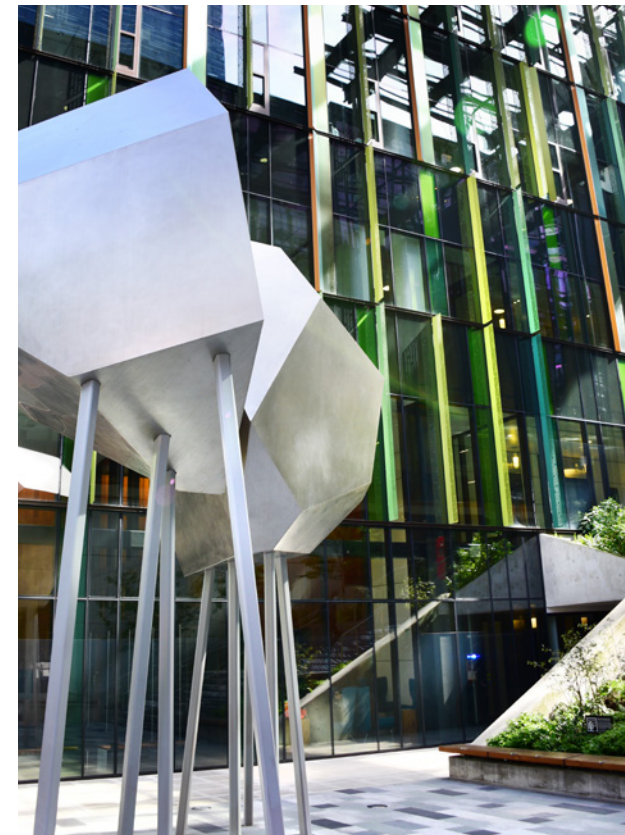
Amazon Doppler tower in Seattle combines sustainable, corrosion-resistant material fits for the coastal location with bright colors on stainless steel by Inox-Color GmbH.
