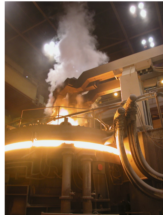
Our operations are energy intensive, but our new energy efficiency target by end of 2024 would mean an energy saving of 600,000 MWh – equal to annual electricity usage of 15,000 households.
