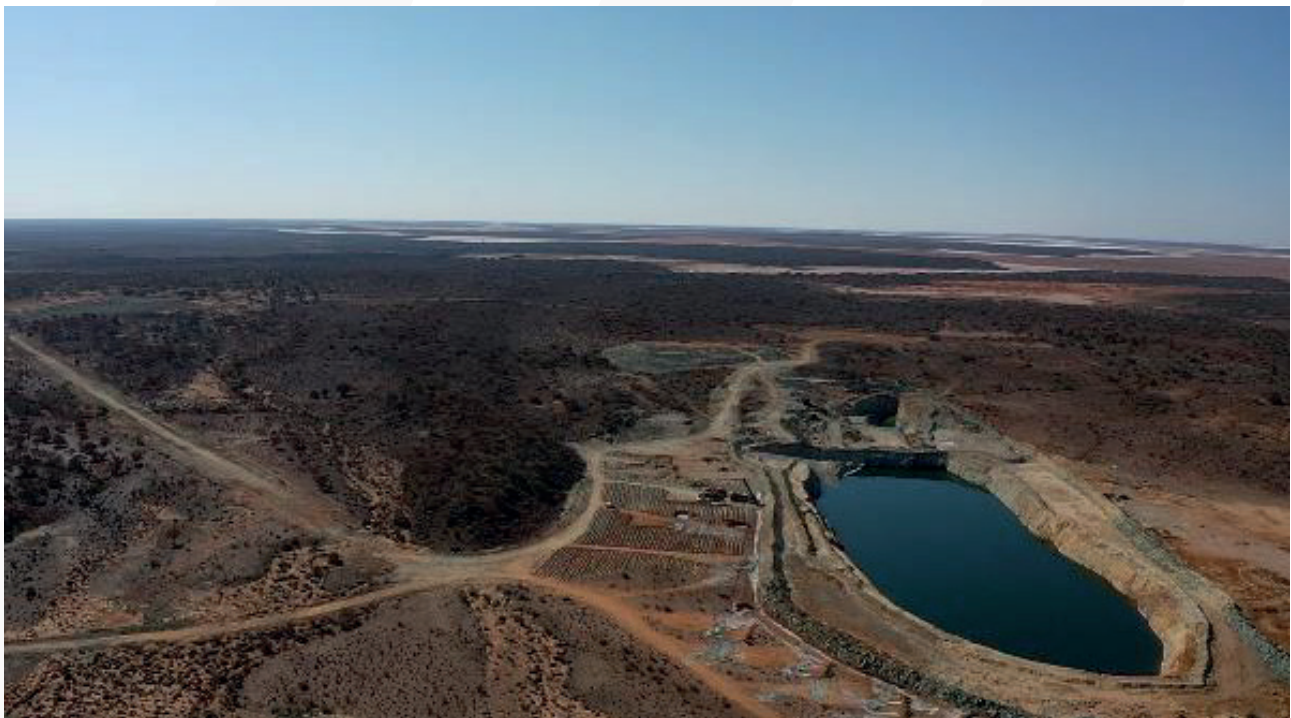
Devon Pit Looking north towards Red October
