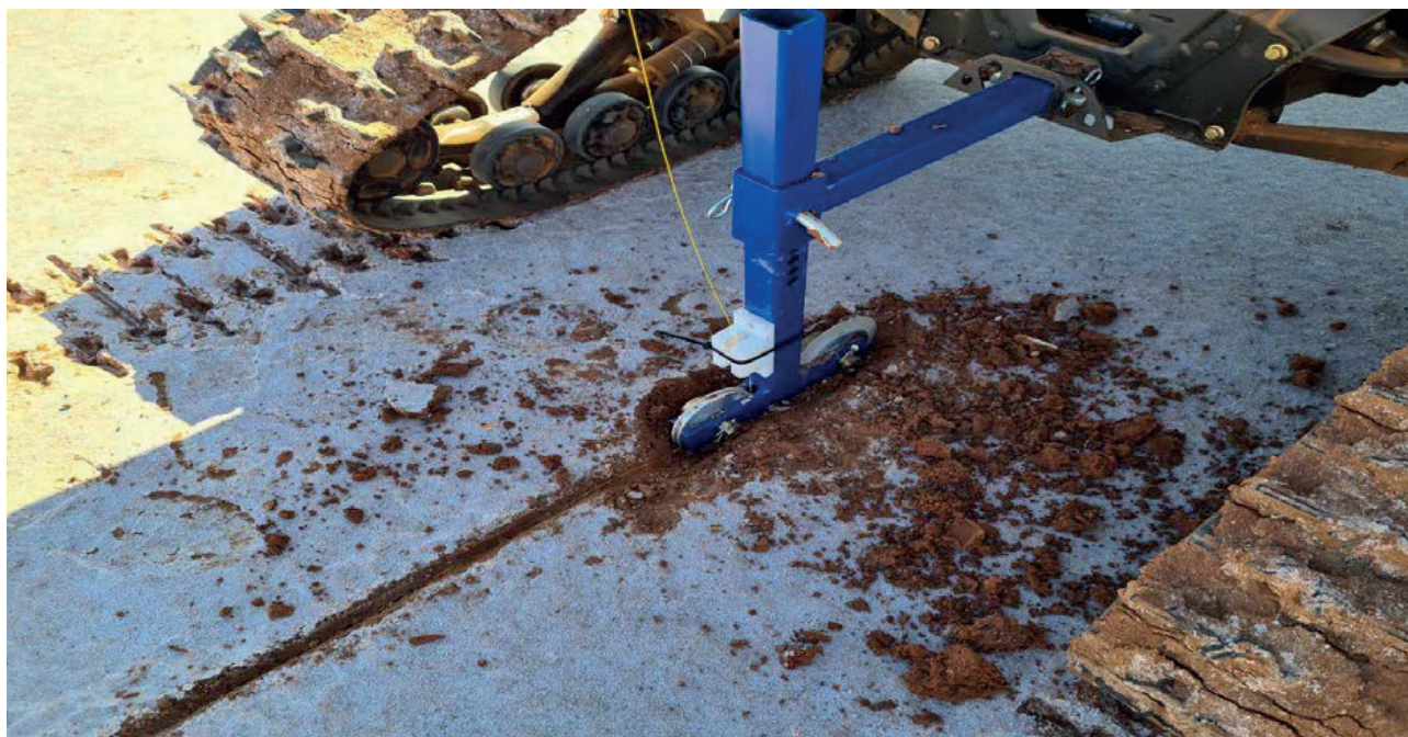
Laying out glass fibre cable at Lake Carey for seismic work
