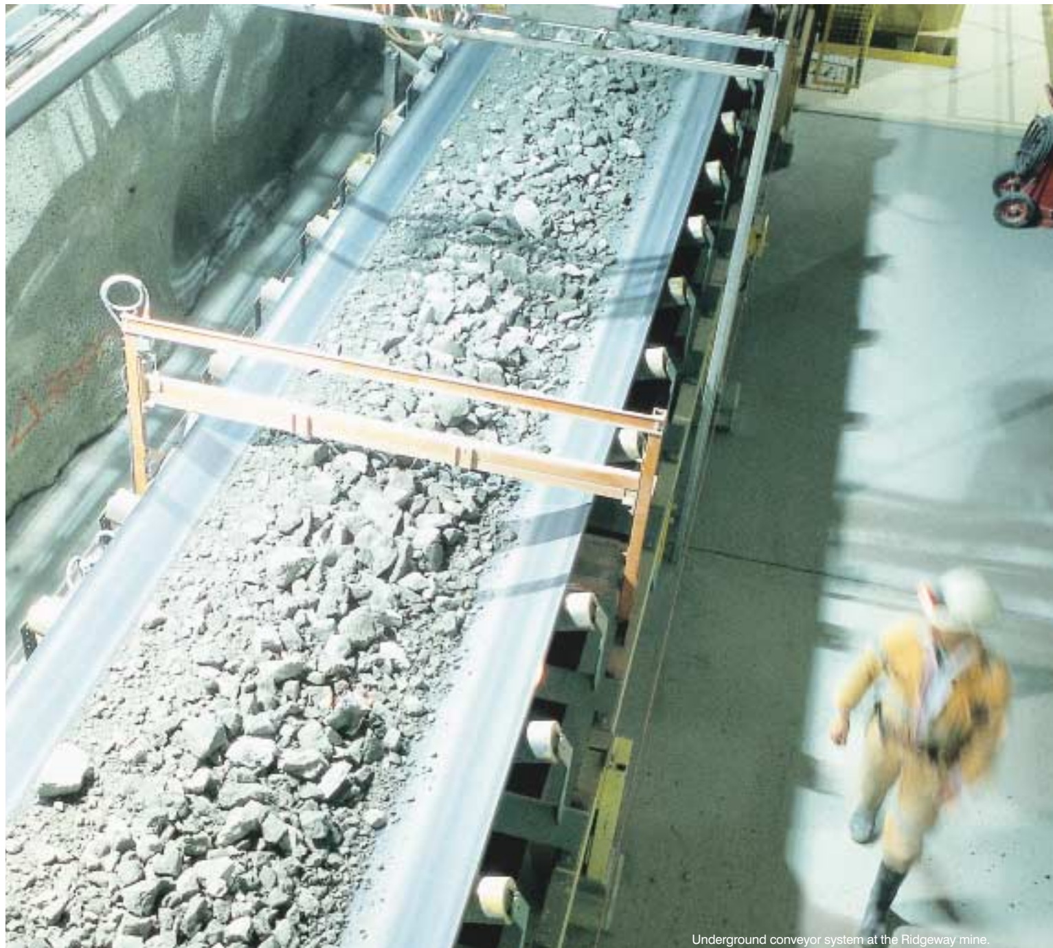
Underground conveyor system at the Ridgeway mine.
