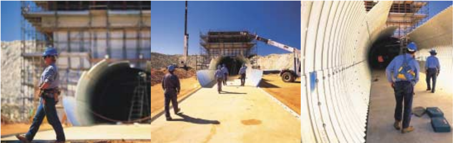
L to R: Construction of Primary Crusher Train 2 – Telfer
