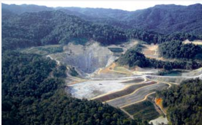
Toguraci Mine showing current Damar pit and backfilled Midas pit (background), with waste dumps (foreground) under progressive reclamation back to the original landform.
