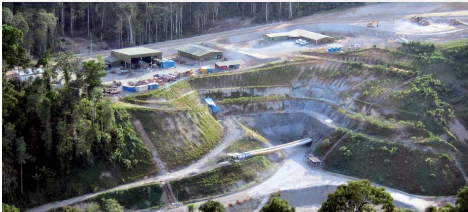
Kencana underground mine portal and ventilation shafts.
