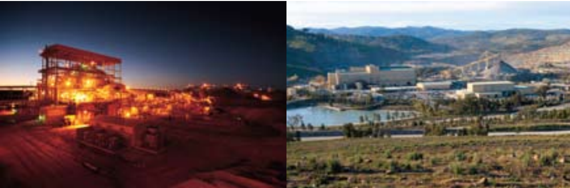
Left Telfer Processing Facility
