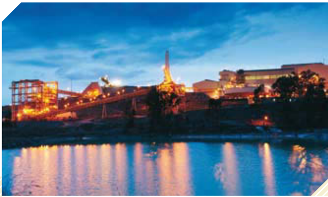
Cadia Valley Processing Plant
