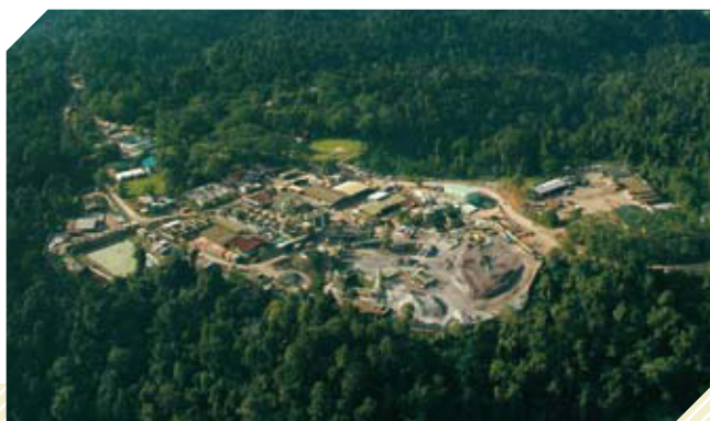
Gosowong Mine Site
