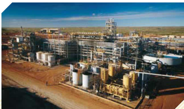
Telfer Processing Plant
