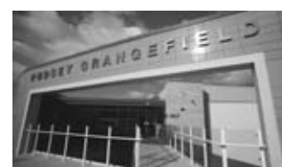
Pudsey Grangefield Maths and Computing College – one of the first BSF schools in Leeds
