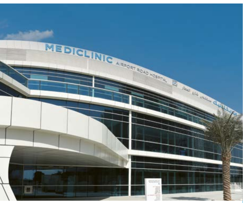
New expansion at Mediclinic Airport Road Hospital, the UAE
