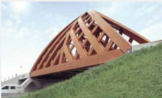
The first of two heavy road traffic bridges in Sneek made from Accoya
