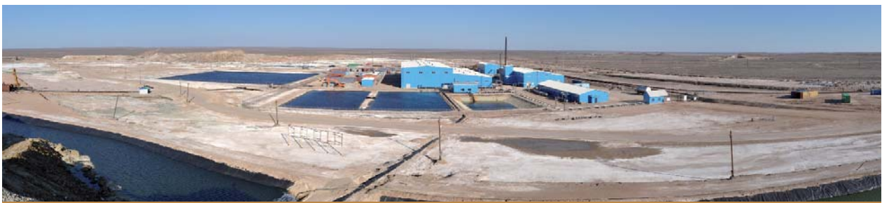
Upper showing Kounrad site prior to construction and lower, April 2012
