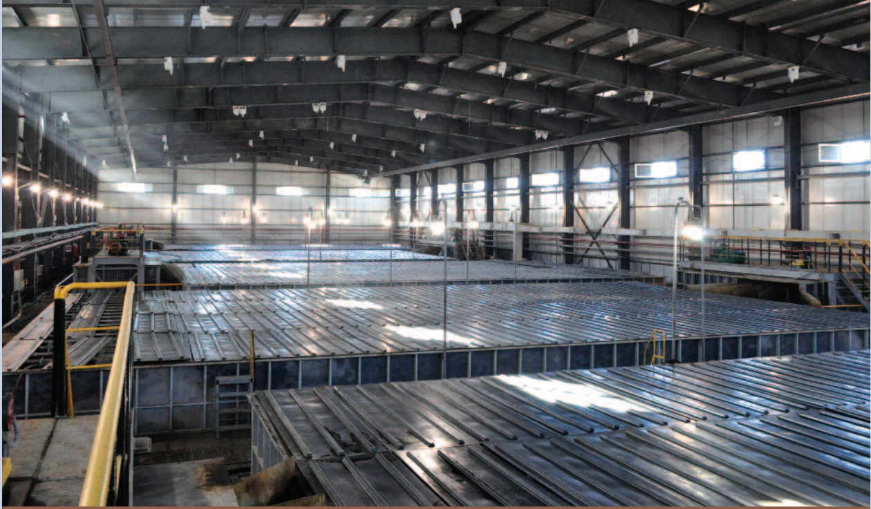
SX building – Kounrad
