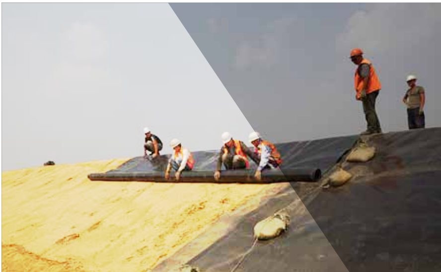
Laying HDPE in new collection trench
