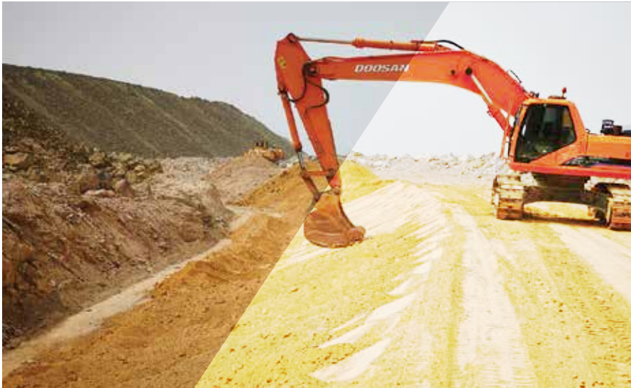
Collection trench construction
