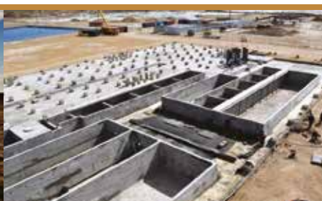
→ 2011 SX-EW construction $39m – $8m under budget
