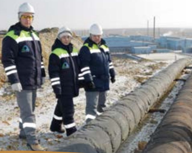
Inspecting solution transfer pipes on the Eastern Dumps
