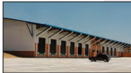
New distribution center—Johannesburg, South Africa
