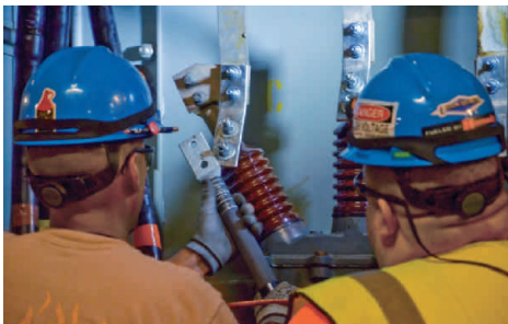
U.S. DEPARTMENT OF ENERGY GASEOUS DIFFUSION PLANT PADUCAH, KENTUCKY
