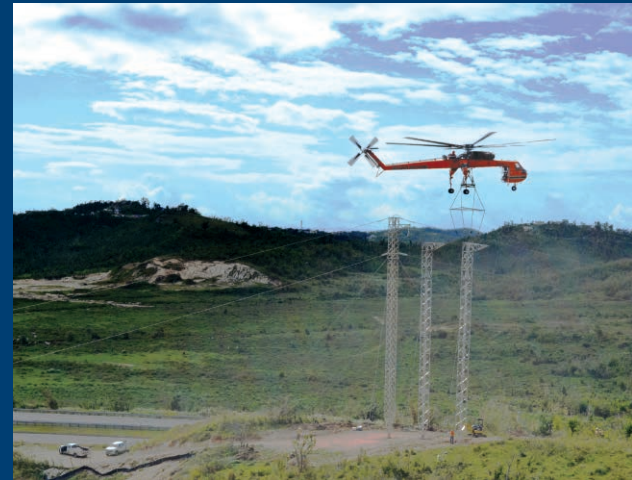
USACE PUERTO RICO POWER RESTORATION — PUERTO RICO
