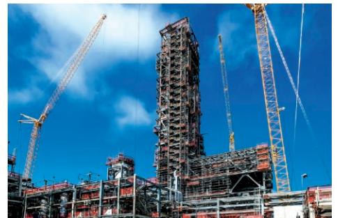
SASOL ETHANE CRACKER AND DERIVATIVES PROJECT WESTLAKE, LOUISIANA — USA
