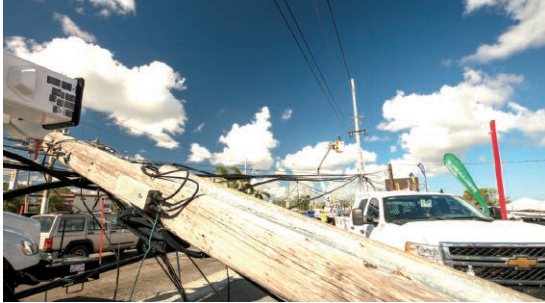
USACE PUERTO RICO POWER RESTORATION — PUERTO RICO
