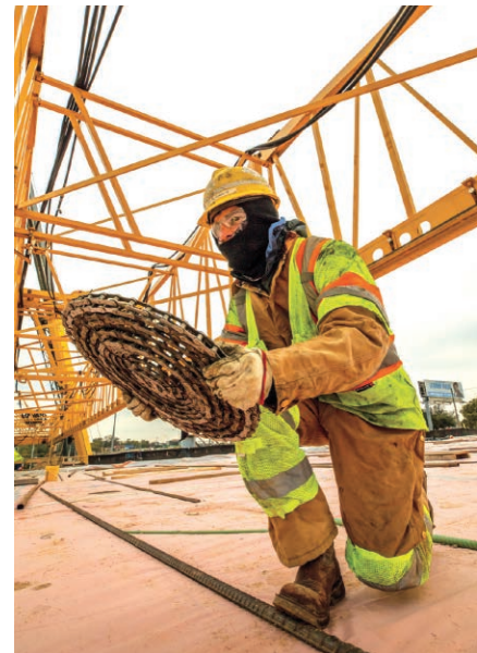
TEXAS DEPARTMENT OF TRANSPORTATION SOUTHERN GATEWAY DALLAS, TEXAS — USA
