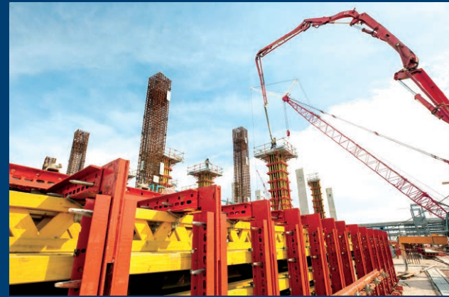
PETRONAS REFINERY AND PETROCHEMICAL INTEGRATED DEVELOPMENT (RAPID) JOHOR – MALAYSIA
