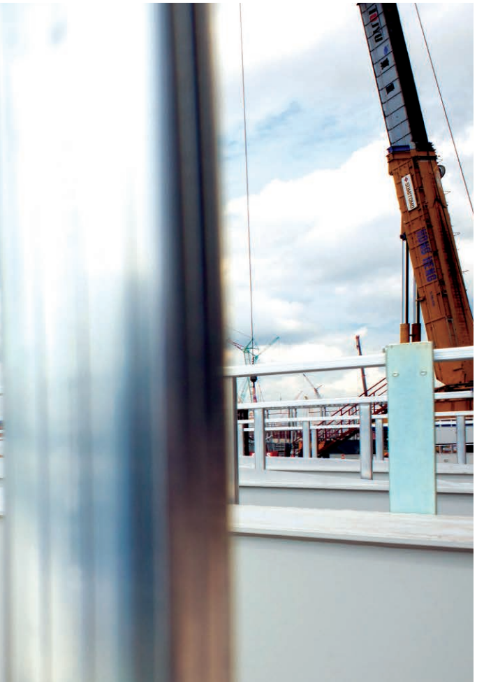
PETRONAS REFINERY AND PETROCHEMICAL INTEGRATED DEVELOPMENT (RAPID) JOHOR — MALAYSIA
