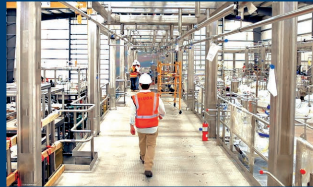
GRIFOLS NORTH FRACTIONATION BIOTECH FACILITY-EPC CLAYTON, NORTH CAROLINA – USA
