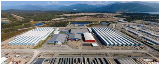
▲ LNG CANADA EXPORT FACILITY KITIMAT, BRITISH COLUMBIA, CANADA
