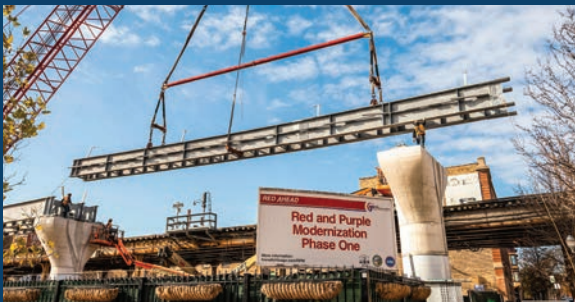
▲ CTA RED AND PURPLE LINE MODERNIZATION PROGRAM CHICAGO, IL, U.S.
