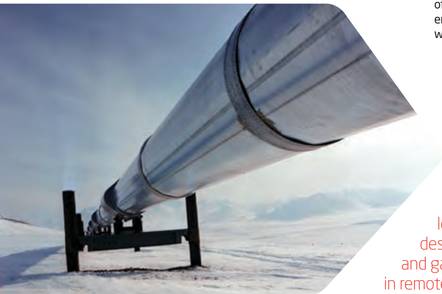
TRANS-ALASKA PIPELINE SYSTEM, ALASKA
