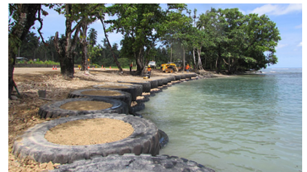
Lipuko Beach after expired mine truck tyres were used to protect the coastline from erosion.
