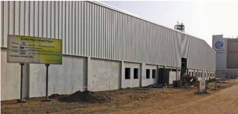
Bonar Natpet facility under construction, Yanbu, Saudi Arabia
