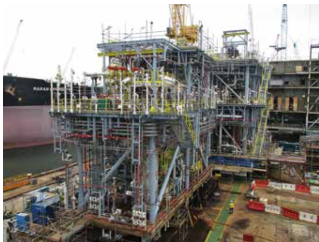
'Energean Power' topsides construction, Admiralty Yard, Singapore
