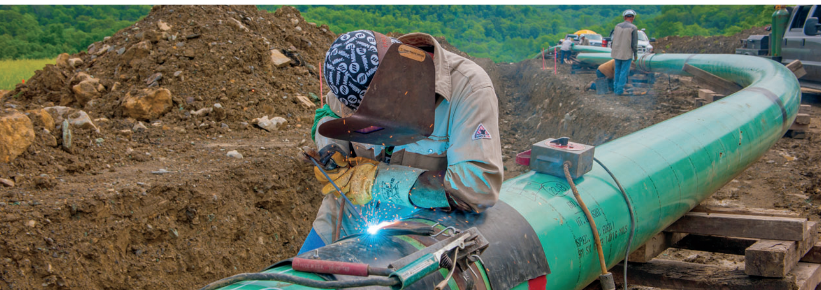
Welding Cornerstone Pipeline near Cadiz, Ohio
