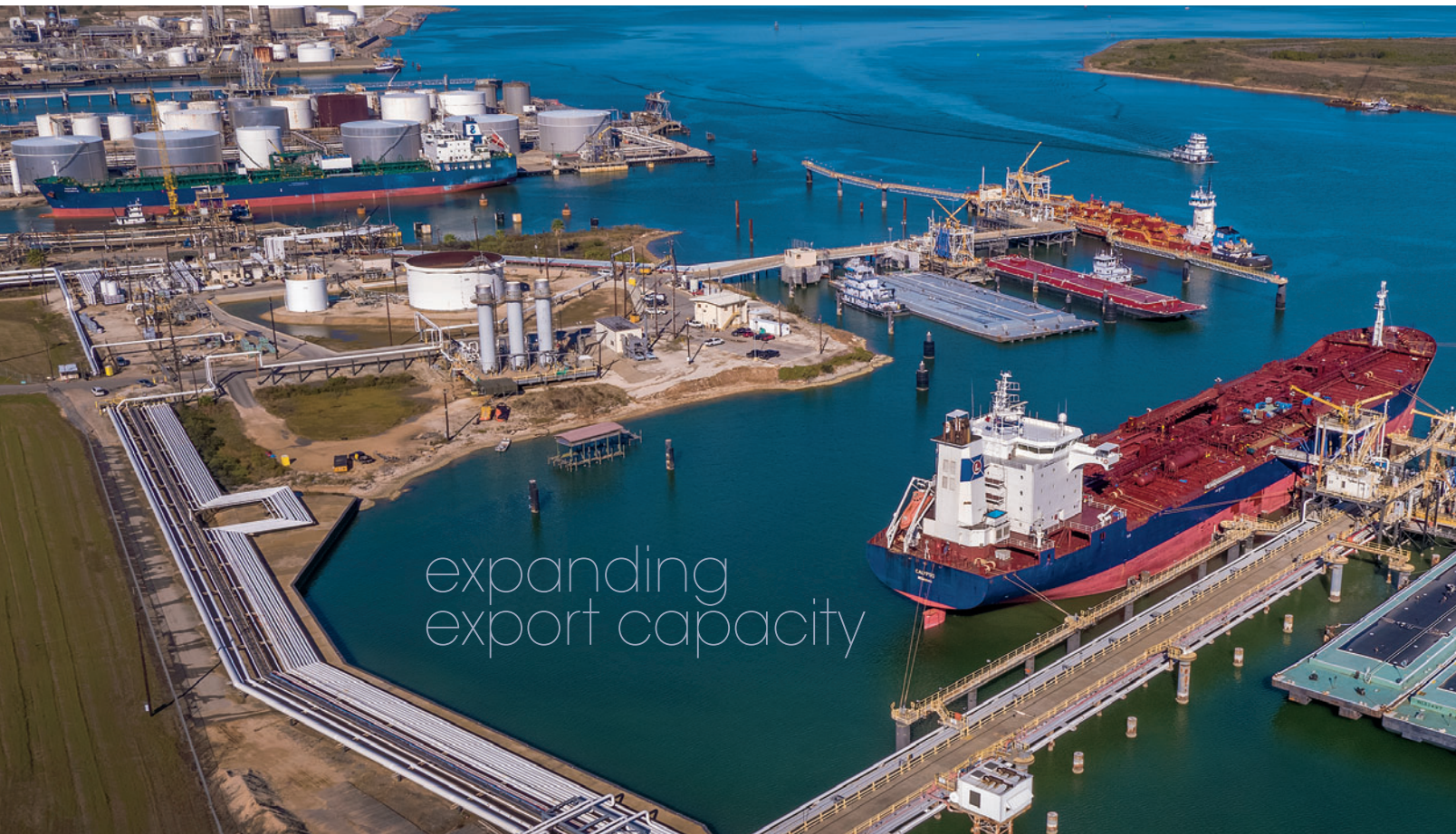
Below: Dock facilities at MPC's Galveston Bay refinery
