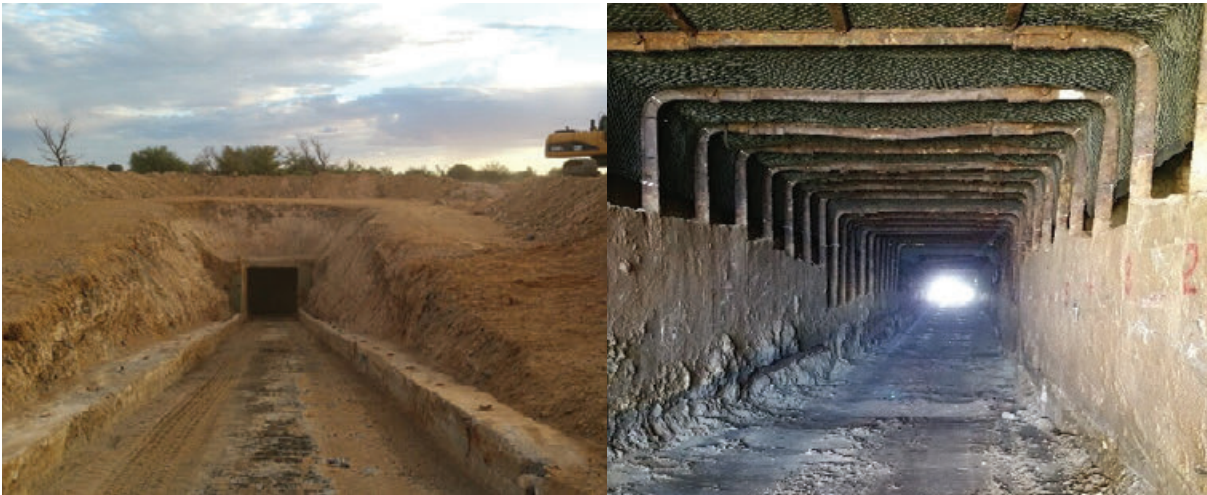
Figure 8: (LHS) Excavating Prieska Project portal (RHS) Rehabilitated decline at Prieska Project portal.
