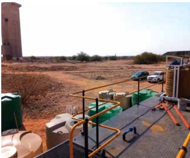
(Left) Water treatment pilot plant mobilisation. (Right) Commissioning the chemical treatment, filtration and reverse osmosis components of the pilot water treatment plant, setup to operate at 5m 3 /hr of feed water.
