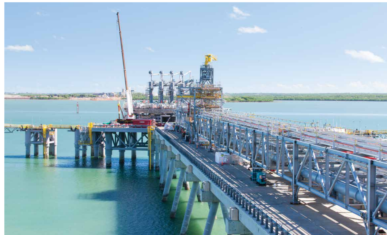
IMAGE Overlooking the jetty at the Ichthys Project Onshore LNG Facilities, Darwin, Northern Territory.
