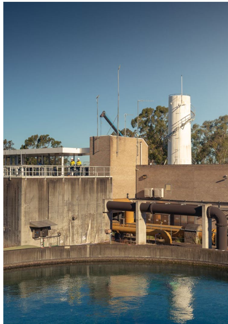
Hunter Water's Dungog Wastewater Treatment Plant in New South Wales.
