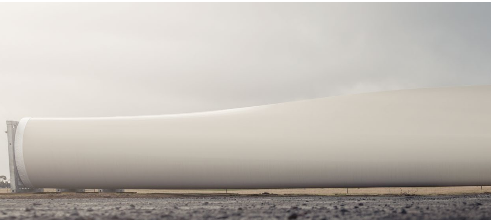
Wind turbine blade ready for erection at Lal Lal Wind Farm in Victoria.
