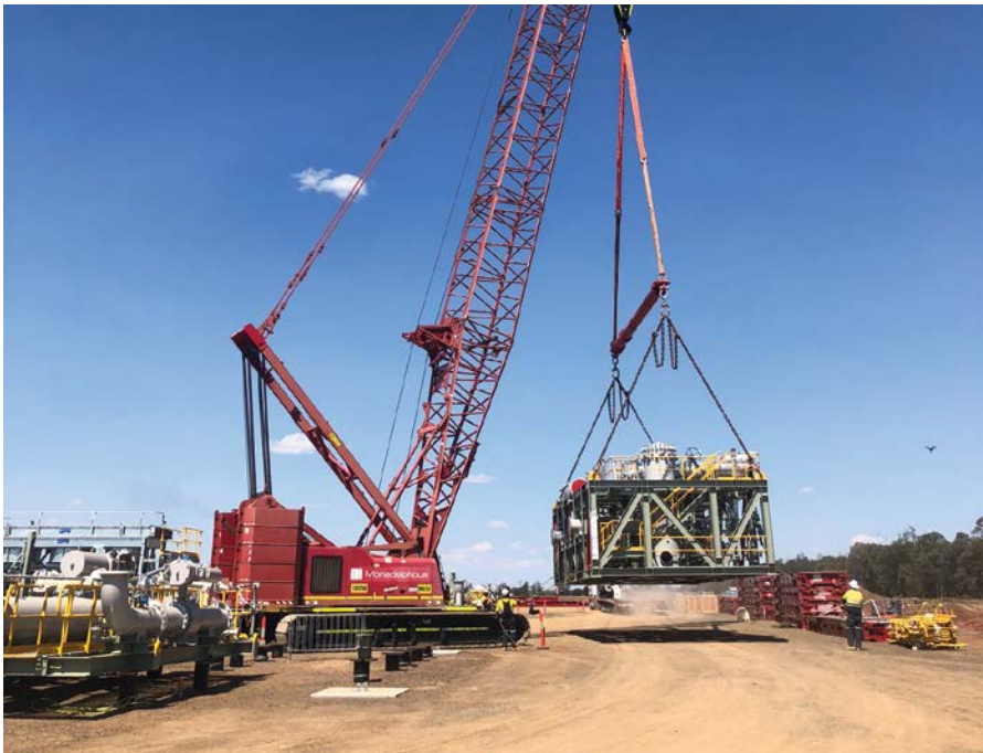
A 250 tonne crawler crane unloading module 153 at Origin's Talinga Orana Gas Gathering Station, Chinchilla, Queensland.
