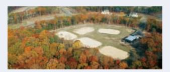
Wastewater is treated through a membrane bio-reactor process which treats water to a high level effluent quality. Effluent is disposed through rapid infiltration basins, a land based disposal alternative that recharges aquifers and ensures groundwater is a renewable resource for future generations.
