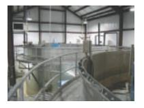
An example of a sequential batch reactor tank operating in Delaware which processes 51,000 gallons of wastewater per day.
