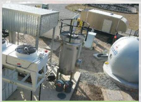
Progress continues on the installation and integration of various components of the anaerobic digestion system at the Ridgewood, NJ wastewater treatment plant.
