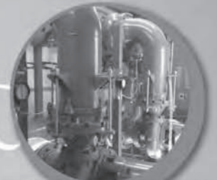
Booster Station Improvements
