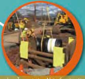
Secondary Transmission Main Construction
