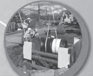
Secondary Transmission Main Construction
