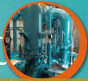
Booster Station Improvements
