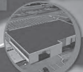
Water Treatment Plant Upgrades
