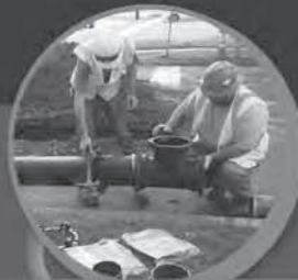
Water Main Replacement
