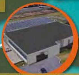
Water Treatment Plant Upgrades
