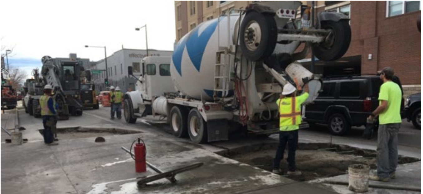
Figure 3. EdenCrete® Trial Slabs on in Denver, Colorado.
