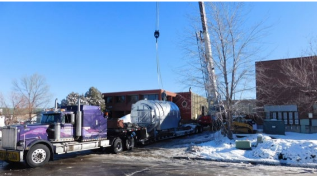
Figure 1. Reactor Being Lifted off Low Loader.
