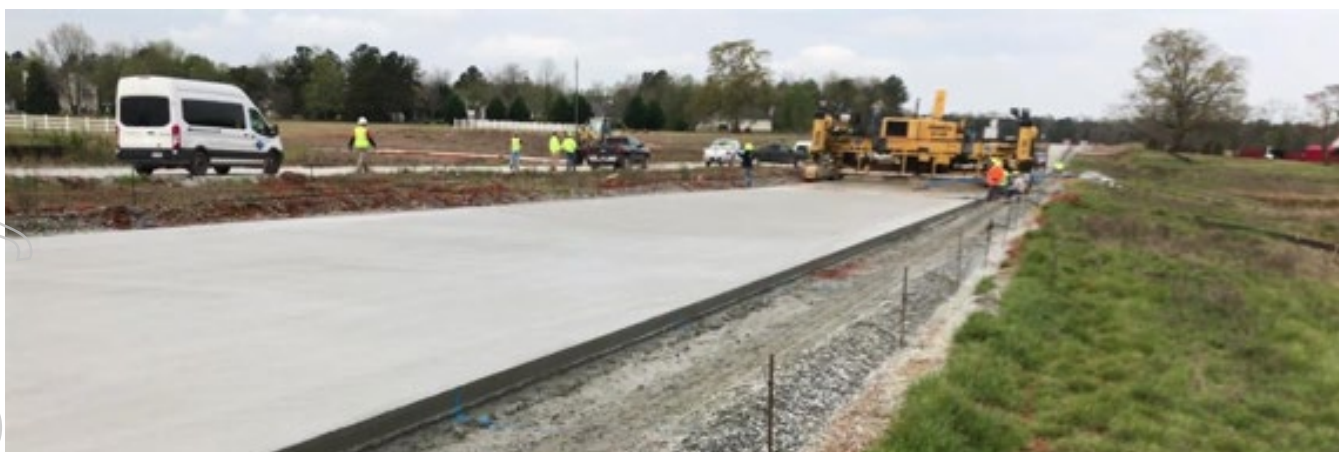
Figure 5. Completed section of highway with added EdenCrete
