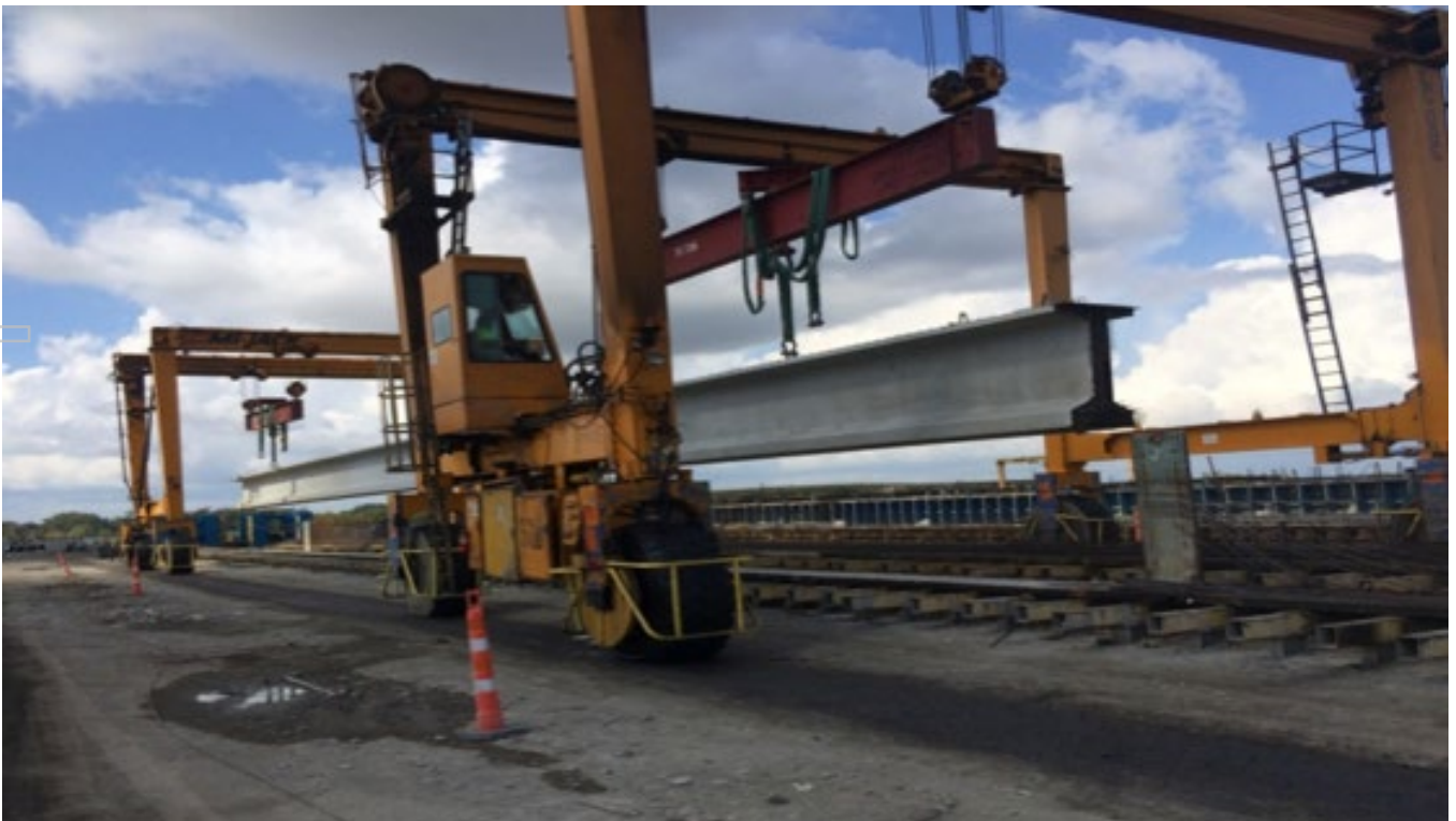
Figure 6. Typical prestressed bridge beam being fabricated at Valley Prestress Products
