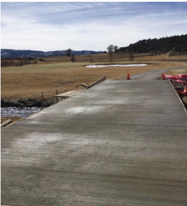
Figure 3. Gypsum Golf Course Bridge Project
