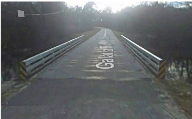
Figure 4. Bridge used for North Carolina DOT trial
