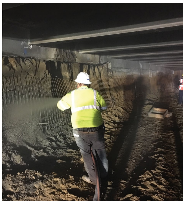
Figure 1. EdenCrete® shotcrete concrete mix being applied
