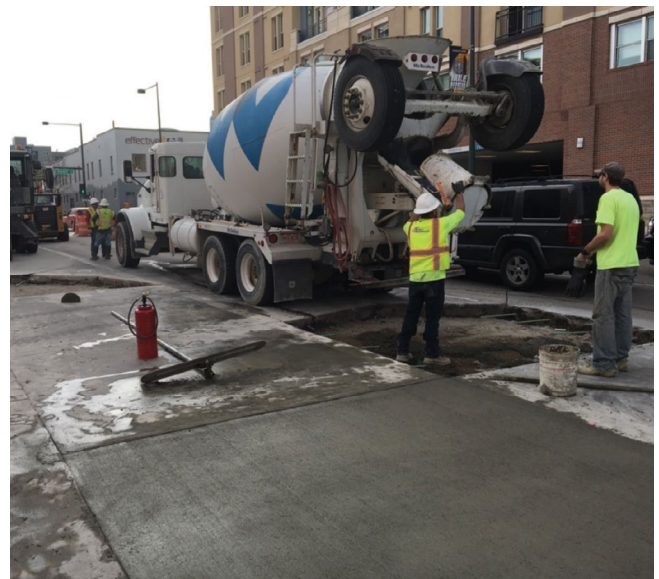
Figure 2. EdenCrete® Trial Slabs in first trials.
