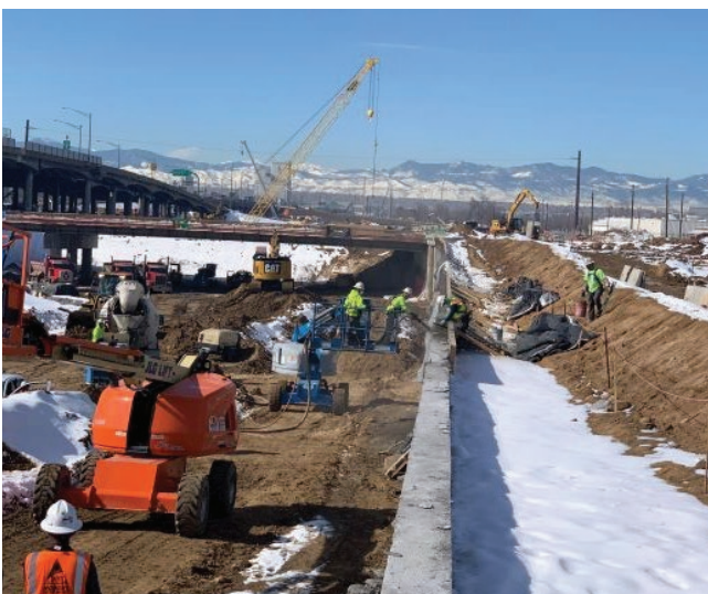
Figure 4. Retaining wall being constructed along Central 70 project using EdenCrete® shotcrete.
