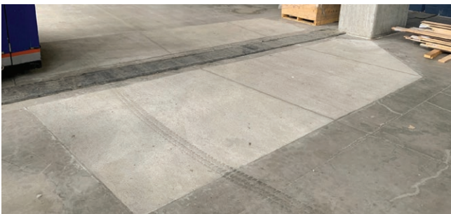
Figure 8. Interior Corridors- 4 inch thick overlay on suspended slab.
