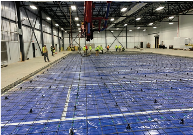
Figure 16. Warehouse floor project for second large company in South Carolina.
