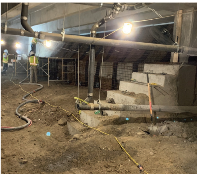
Figure 10. Centres for Health, Nutrition and Physical Therapy- EdenCrete® used in shotcrete for walls.
