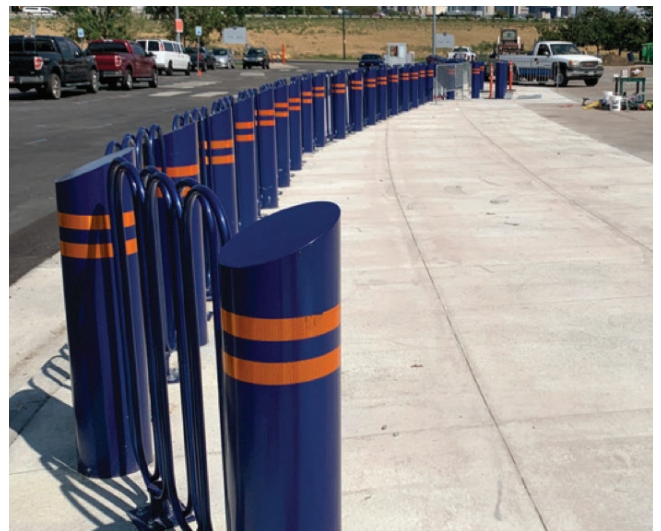
Figure 13. Steel Ballard security Screening Areas - 6 inch thick full-depth slab.
