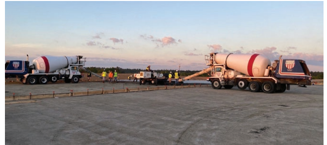
Figure 15. 200,000 square foot Industrial slab being poured.
