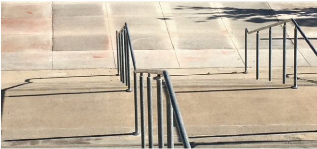
Figure 7. Perimeter Facilities - 5- 6 inch thick, full-depth slab repair.
