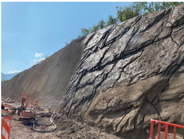
Figure 3. Shotcrete retaining wall being sculpted to look like natural rock face.
