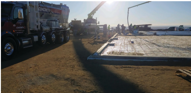
Figure 7. Volumetric truck mixing at the Loveland project site
