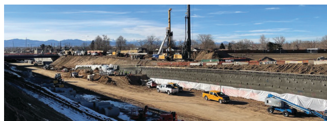
Figure 1. Shotcrete section along Central 70 Project
