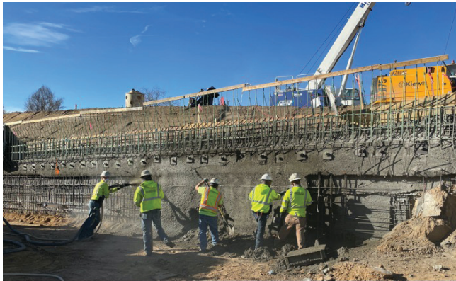
Figure 2. Shotcrete being applied on Central 70 Project
