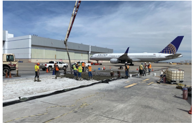
Figure 8. Replacement of concrete panels on United Airlines maintenance hangar apron.
