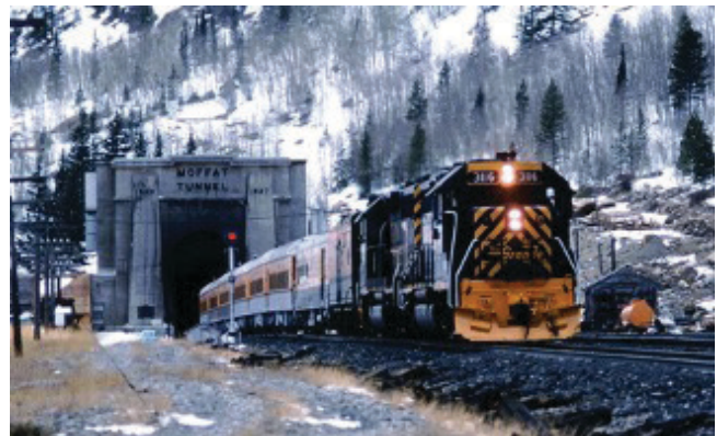
Figure 9. The East Portal of the Moffat Tunnel
