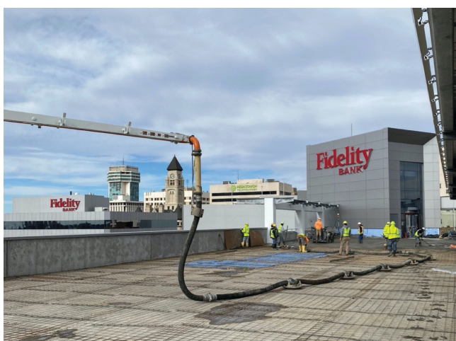
Figure 11. Installing top deck of car park
