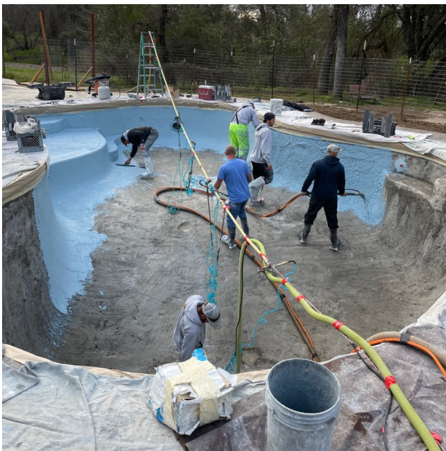
Figure 2. A typical US exposed aggregate, swimming pool finishing mix being applied.
