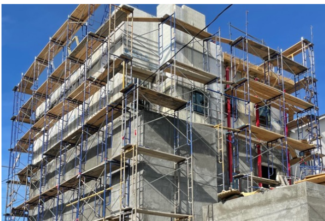
Figure 7. 4-storey SCIP residential home in Houston under construction and including EdenCrete®
