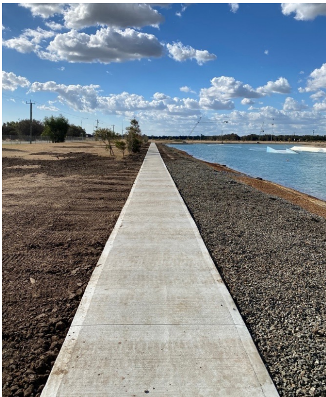
Figure 9 Concrete pavement (including EdenCrete®) at Perth Wake Park
