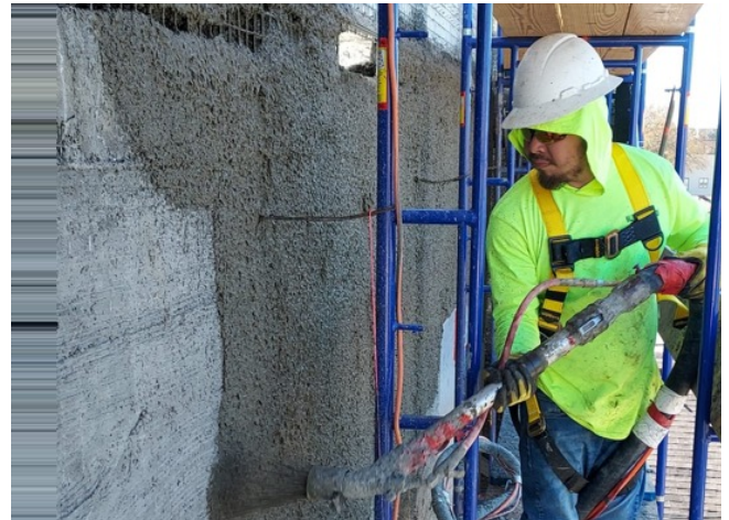
Figure 8. Shotcrete mix with EdenCrete® filling and fully encapsulating the wire mesh
