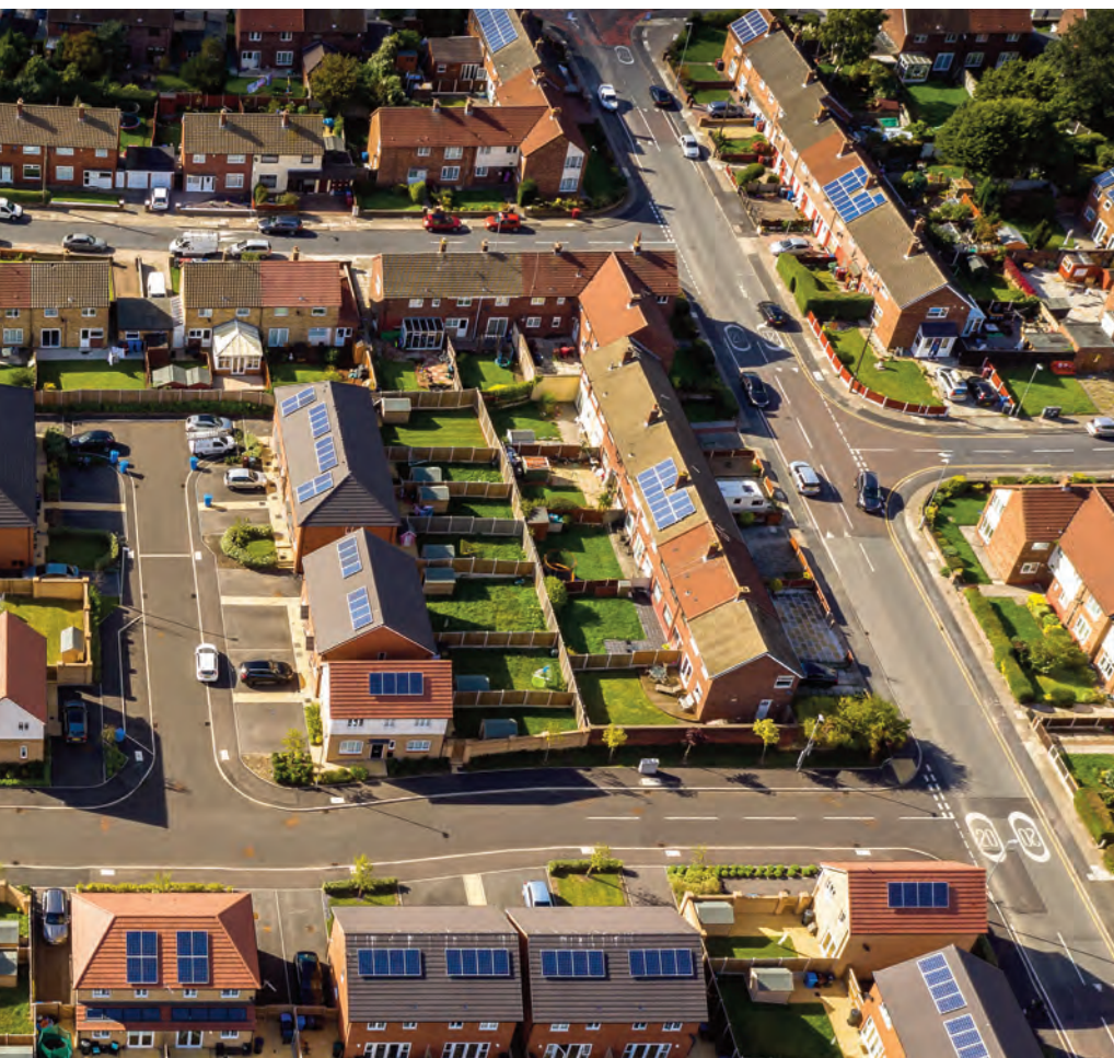
Aerial view of Woodbine Road, Halewood
