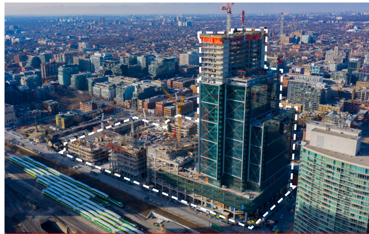
▶ The Well™ Development Progress | Toronto
