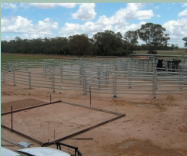
A set of cattle yards recently constructed on Woodlands. A curved structure such as this assists the movement of the cattle and reduces the chances of stress or injury.
