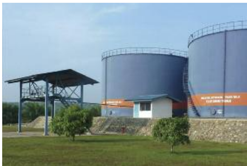
Crude-palm-oil storage tanks at the Pangkatan mill.
