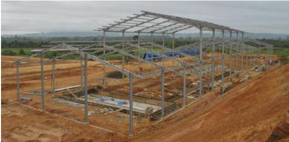
New mill building taking shape on the Kalimantan project.
