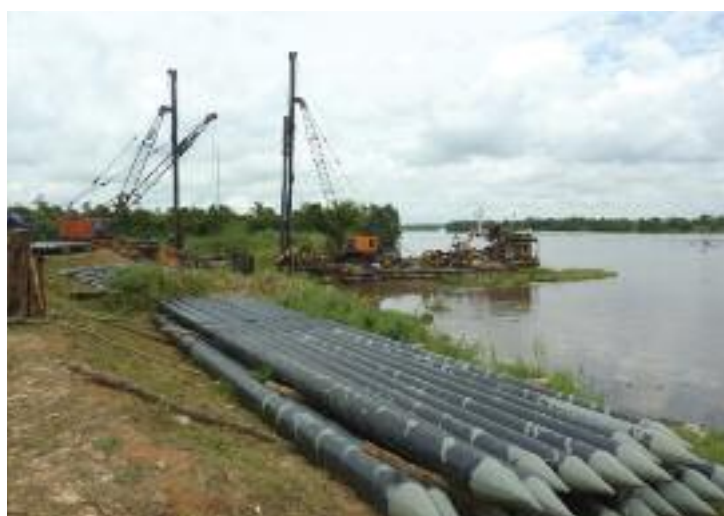
Piling for the new jetty in Kalimantan.
