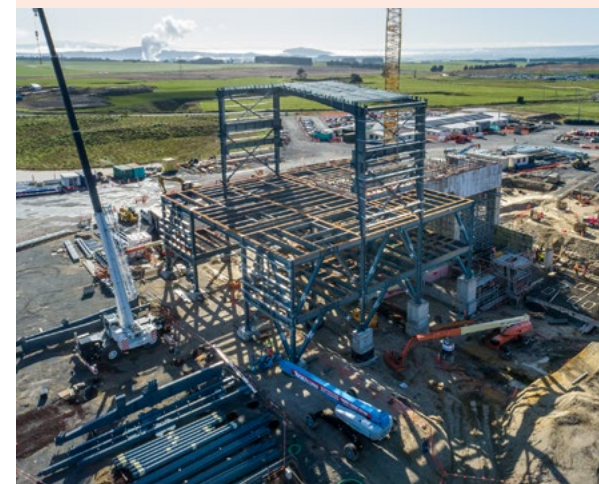
Progress on the turbine hall of Tauhara Power Station.
